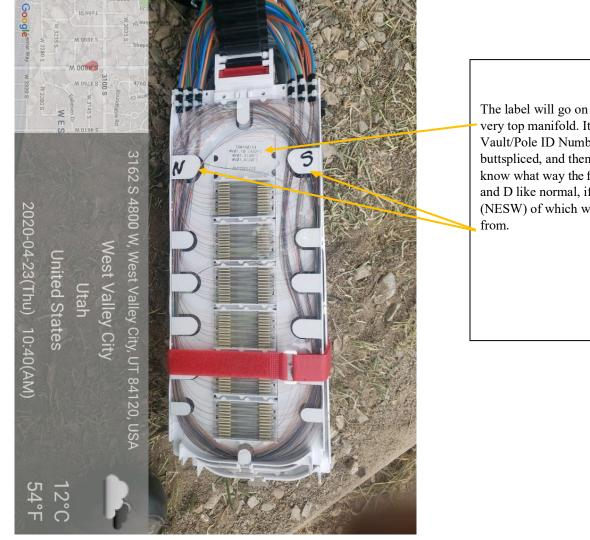
The label will go on the tray itself in the very top manifold. It needs to include Vault/Pole ID Number, then cable(s) being buttspliced, and then BUTTSPLICE. If you know what way the feed comes from, put F and D like normal, if not, use directions (NESW) of which way the cable(s) come from.
